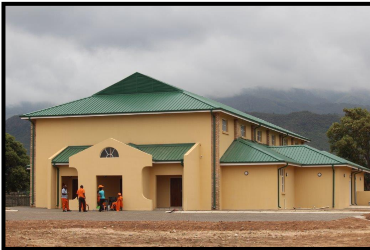
Moshate Community Hall
